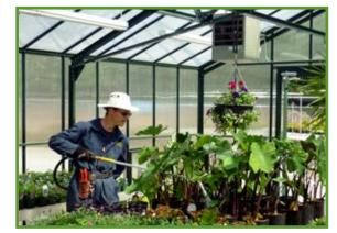
A twinwall polycarbonate greenhouse illustrating that glazing is not a transparent product and only shapes are visible.
